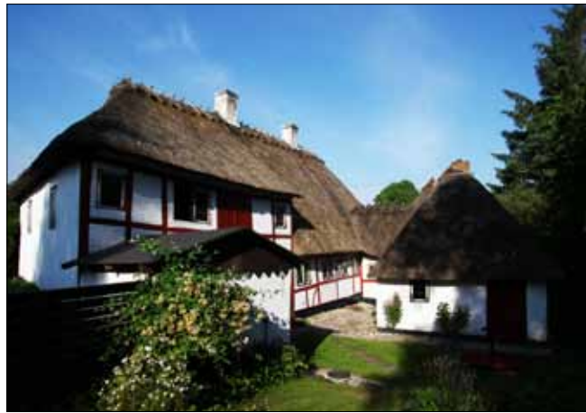
From the garden you can see the very special building and, in addition, the old well.
